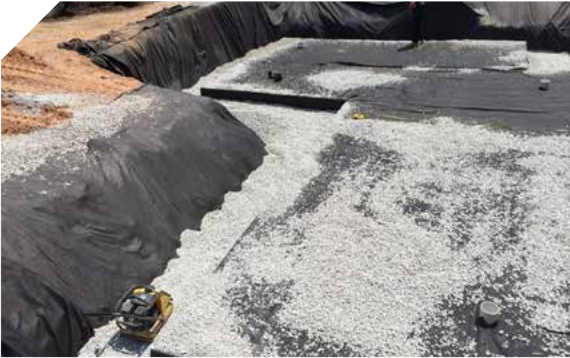
Correctly Backfilled
